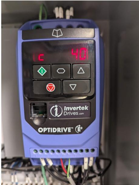
Inverter VFD - Press the Octagon to scroll through
