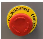
Emergency Stop switch located on the side of the electrical box
